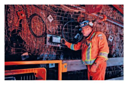
communications solution; a Gigabit network providing both power and data using flexible coaxial cable.
