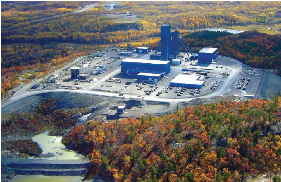
Stantec completes engineering of the underground infrastructure, including ventilation infrastructure, of Nickel Rim South, in Sudbury, Ontario. (Photo: Stantec)
